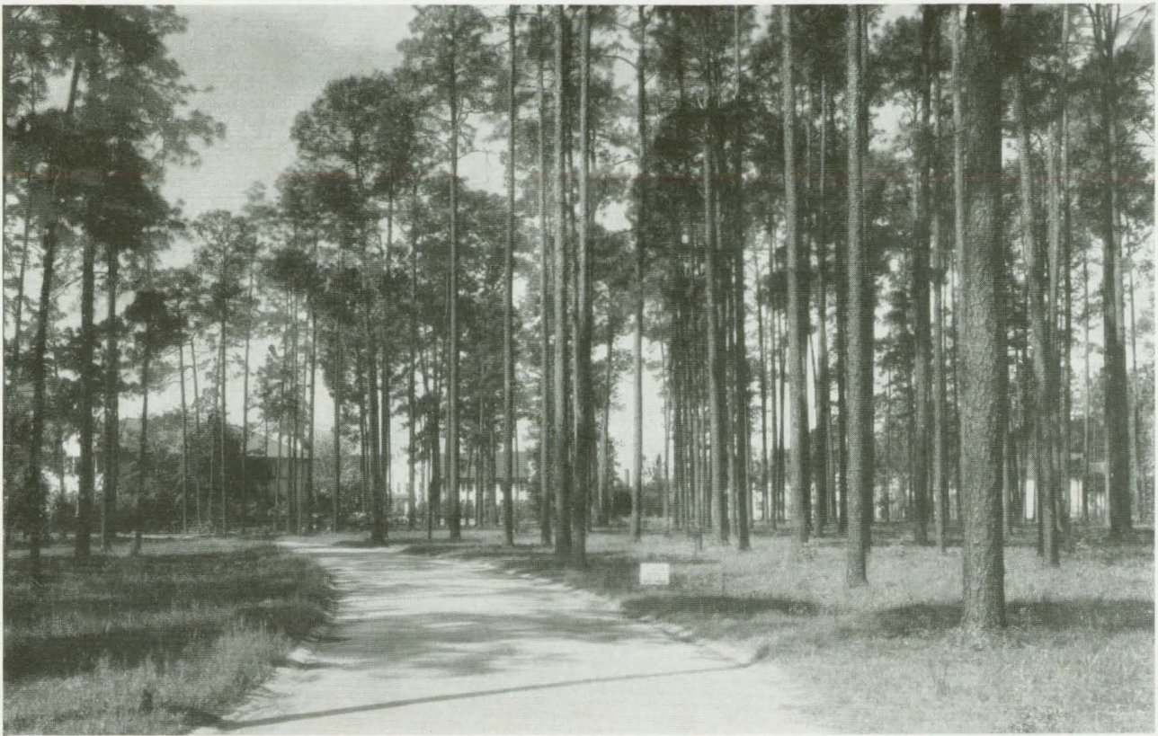
A Mile of Concrete Roadways on the Campus
