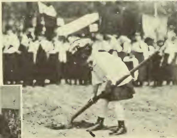
Caroline Parrish (Thomas) Spades First Ground for West Hall (Fall 1916)
