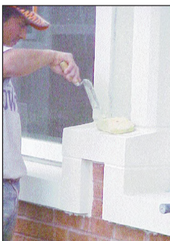
A worker grouts a window ledge at the Rec Center.
