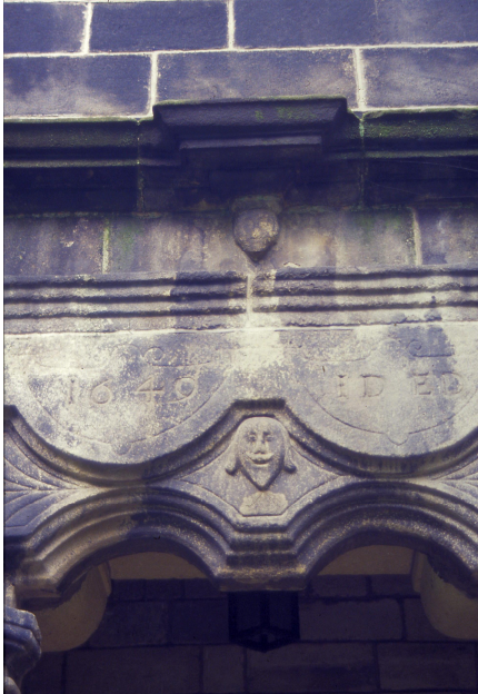
Fig. 1: Wood Lane Hall porch
