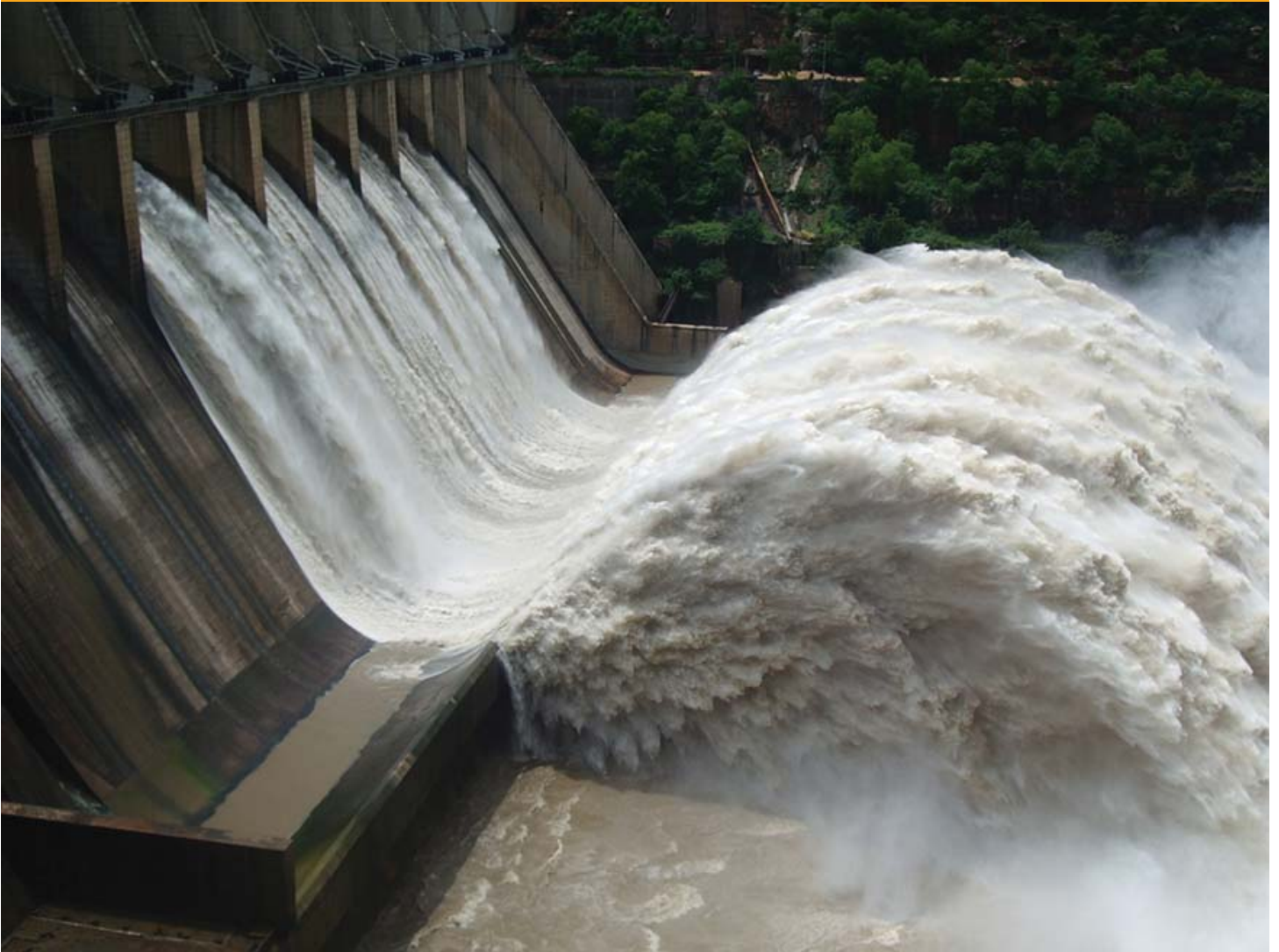
Figure 20.1 Electric energy in massive quantities is transmitted from this hydroelectric facility, the Srisaïlam power station located along the Krishna River in India, by the movement of charge—that is, by electric current. (credit: Chinto here, Wikimedia Commons)
