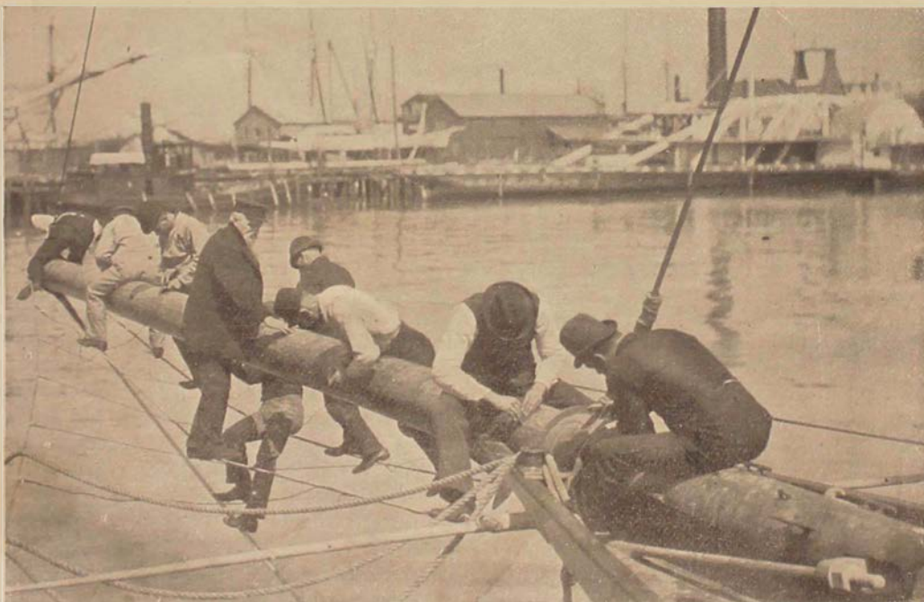
SCRAPING THE BOWSPRIT.
