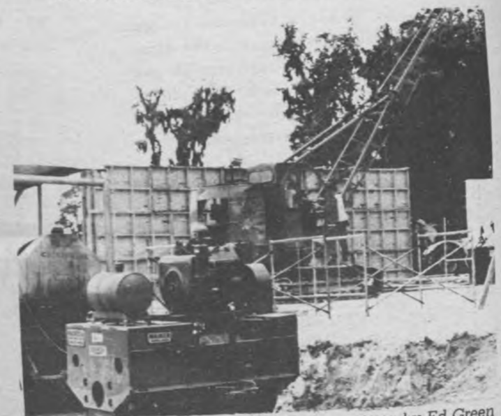
Concrete backboards for tennis courts. photo by Ed Green
