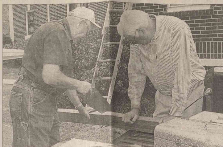
MARCUS SHIERLING, left, contractor and Ray Council, Rayann's Church Furnishings, saw the boards the old way with a hand held saw, to make the rafter braces for inside the Presbyterian Church, to complete installation of steeple.
