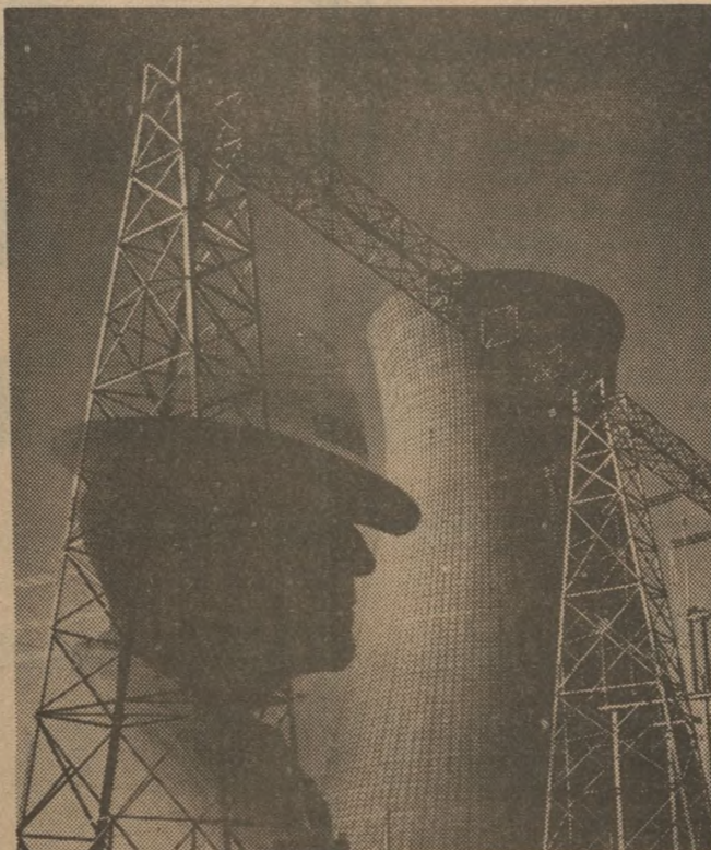
Photographic montage showing one of cooling towers at Plant Bowen.
