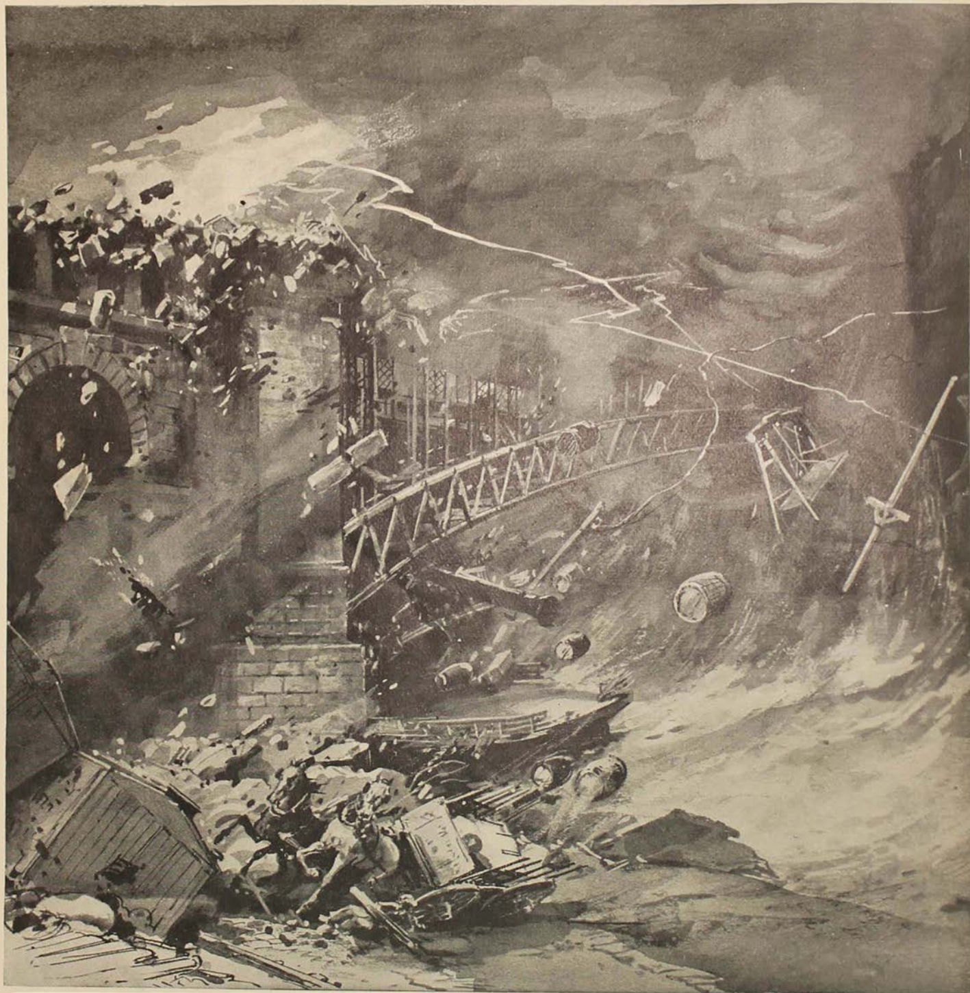
DESTRUCTION AT THE EAST ST. LOUIS END OF THE EADS BRIDGE.
