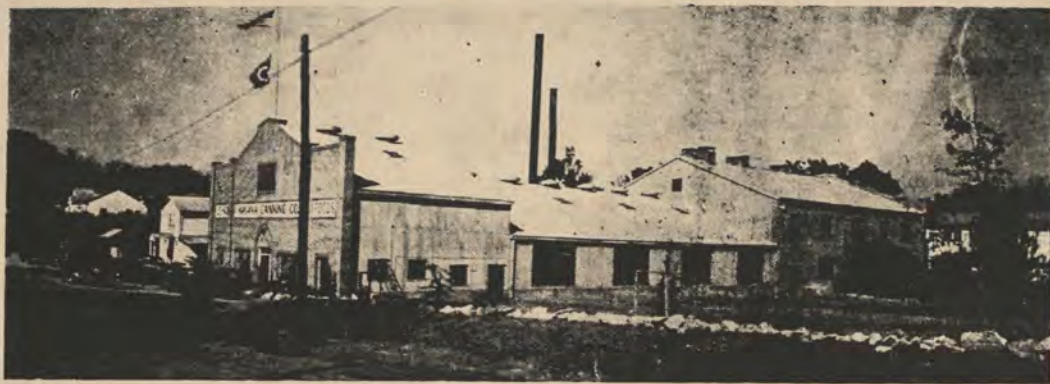
CANNING AND DEHYDRATING PLANT OF HAVANA CANNING CO., COMPLETED IN 1943
