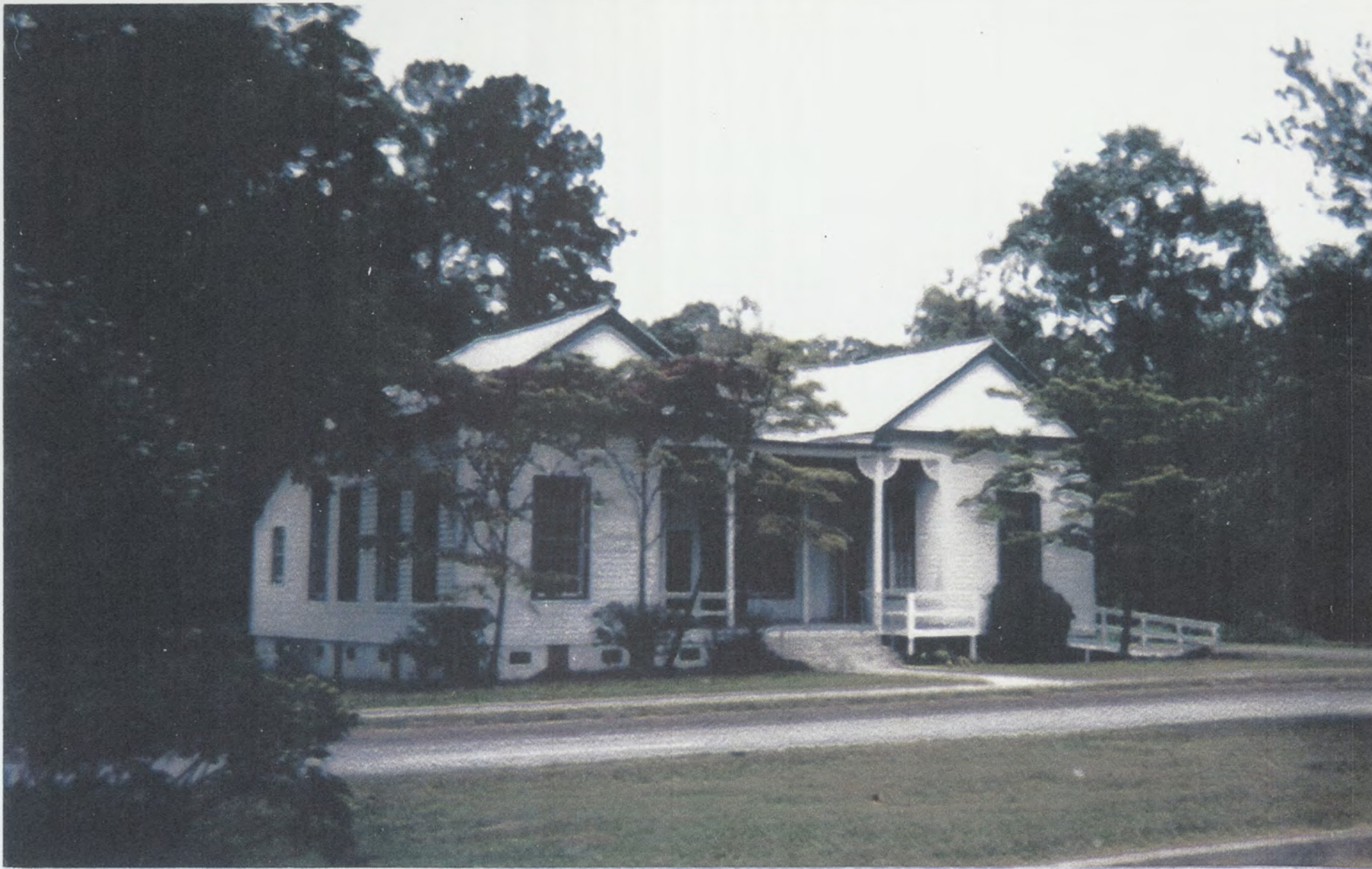
Bentley House – 508 W. Screven Street built in 1860.
