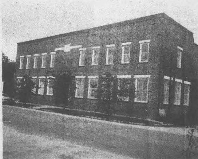
South Ga. Grocery Co. Warehouse and Main Office Building located at S. Washington St., Quitman, Ga.
