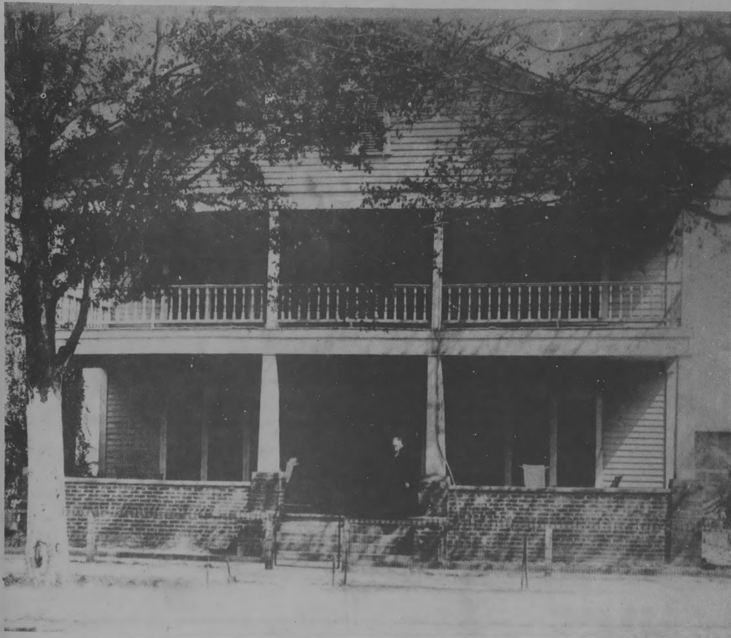
Photo - Courtesy of Norwood Miley THEN BOARDING HOUSE -Mrs. Mattie Massey stands on the porch of the house as it looked after 1914 when she operated it as a boarding house.
