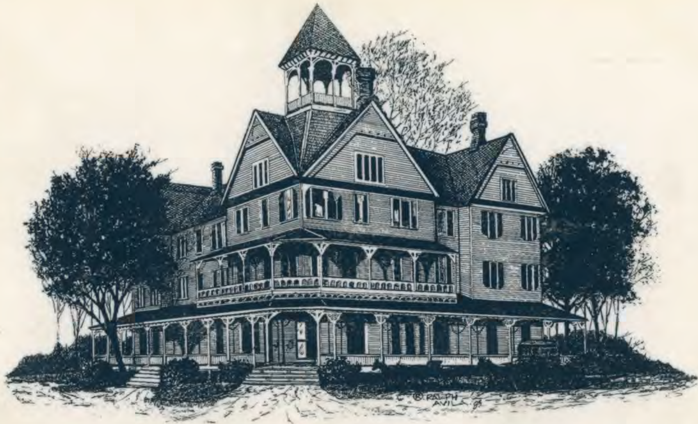
HOTEL MARIE -In 1889 Quitman leaders realized the need for hotel facilities here. F. J. Spain and Henry G. Turner were leaders in a drive to raise funds for construction and $13,000 was collected in a short time. The Quitman Hotel Company was organized and the Purcell lot on Screven Street was purchased for $1,800. A pretentious and unusually large 3 story structure with verandas extending around the building. A. H. Johnston was the architect and S. A. Remington contractor of the 46 room hotel. The hotel company named it Hotel Marie in honor of F. J. Spain's young daughter. The Hotel Quitman is now located on the Hotel Marie site.
