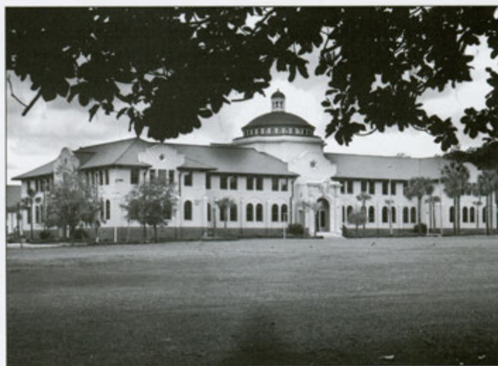
West Hall, located in the center of Valdosta State University's main campus, houses the offices of the president and vice president for academic affairs as well as several academic departments.
