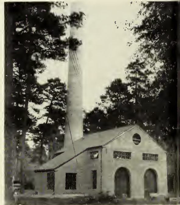
Newest Addition—Heating Unit
