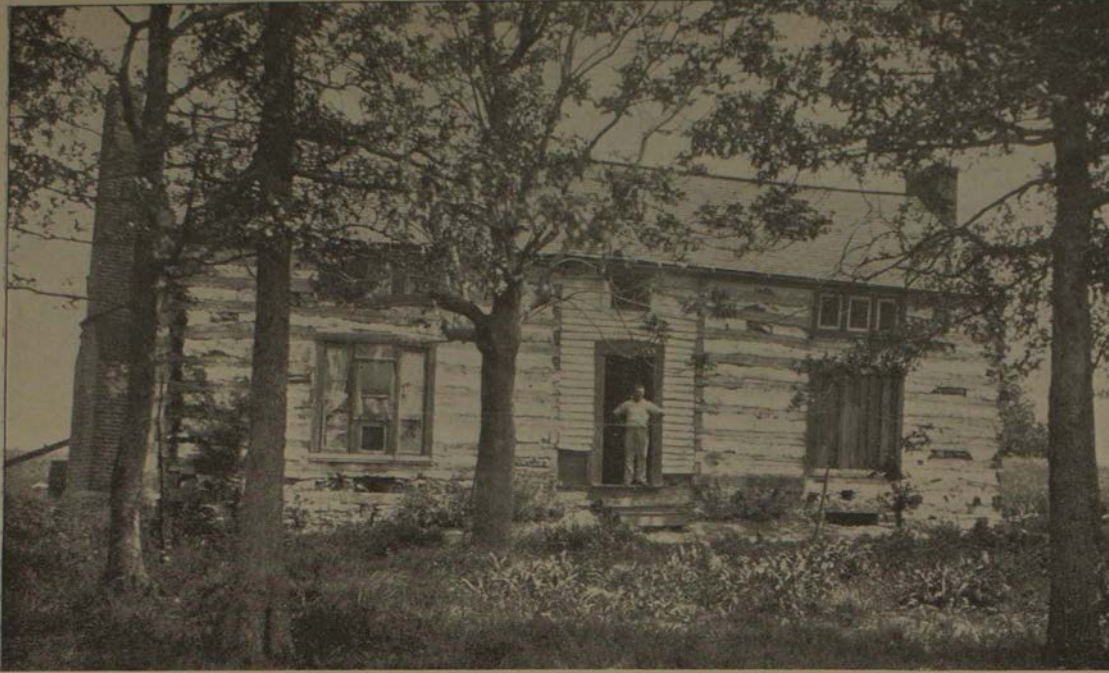
GENERAL GRANT'S OLD HOME IN ST. LOUIS COUNTY, MISSOURI.
