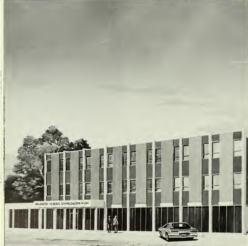
Valdosta Federal Savings And Loan Association
