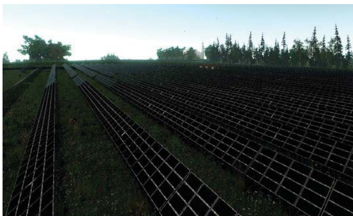
Figure 7.31 Solar cell arrays at a power plant in Steindorf, Germany (credit: Michael Betke, Flickr)
