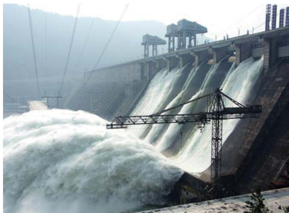
Figure 7.38 Hydroelectric facility (credit: Denis Belevich, Wikimedia Commons)
