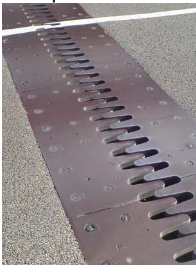
Figure 13.10 Thermal expansion joints like these in the Auckland Harbour Bridge in New Zealand allow bridges to change length without buckling. (credit: Ingolfson, Wikimedia Commons)
