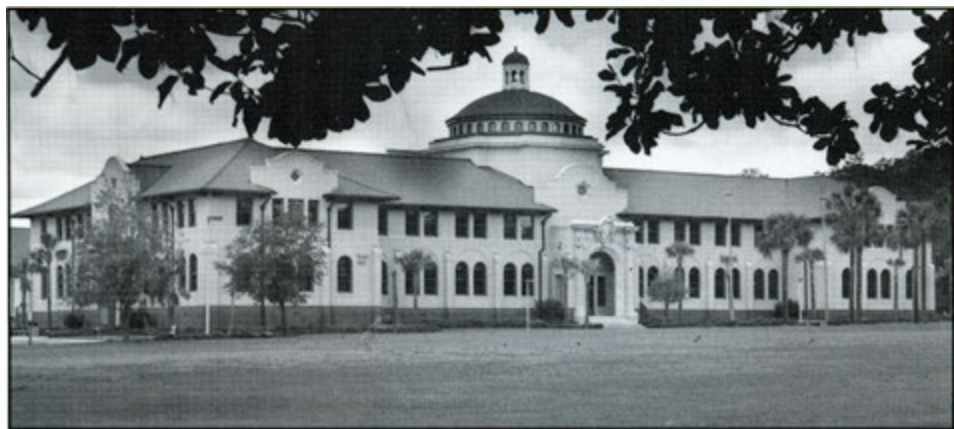
West Hall, located in the center of Valdosta State University's main campus, houses the offices of the president and vice president for academic affairs as well as several academic departments.
