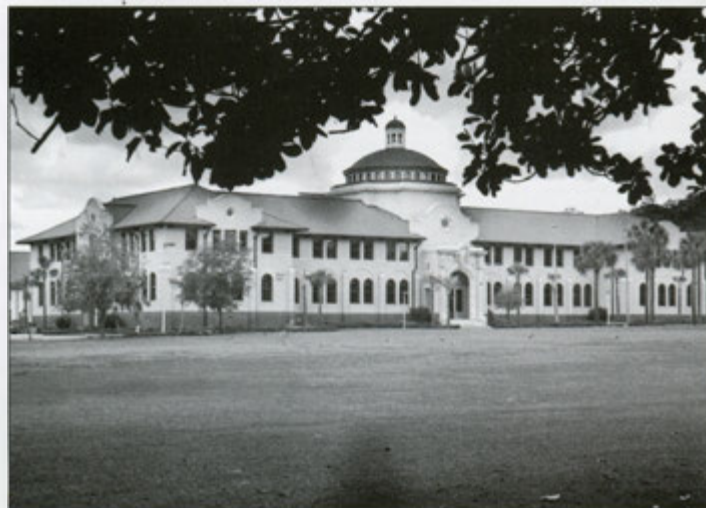
West Hall, located in the center of Valdosta State University's main campus, houses the offices of the president and vice president for academic affairs as well as several academic departments.
