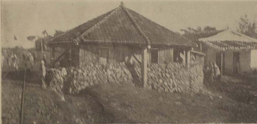
STONE FORT ON HAVANA STRONG LINE.
