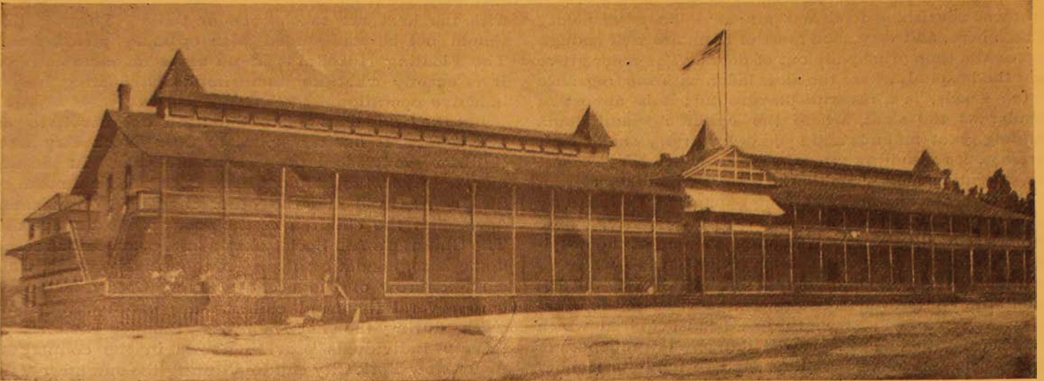
THE SEASIDE HOSPITAL BUILDING, CEDAR GROVE, STATEN ISLAND.
