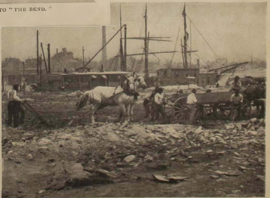
BREAKING GROUND FOR THE PARK AT CORLEAR'S HOOK.
