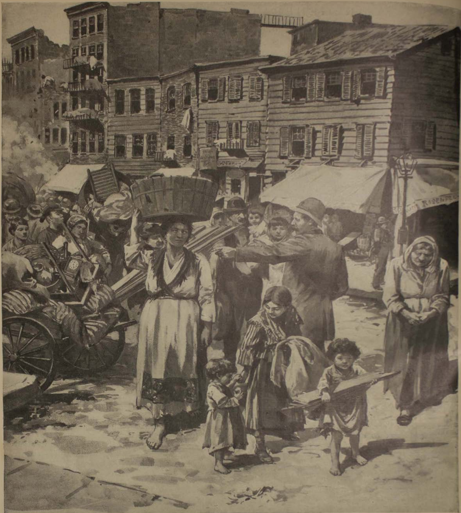
MOVING OUT OF MULBERRY BEND PREPARATORY TO THE CONSTRUCTION OF THE NEW PARK.
