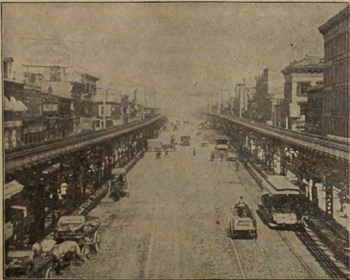
THE ELEVATED RAILWAY ON THE BOWERY.
