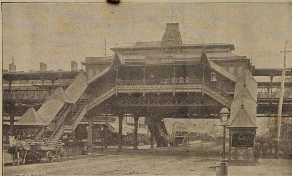
STATION OF THE ELEVATED RAILWAY AT FOURTEENTH STREET AND SIXTH AVENUE.
