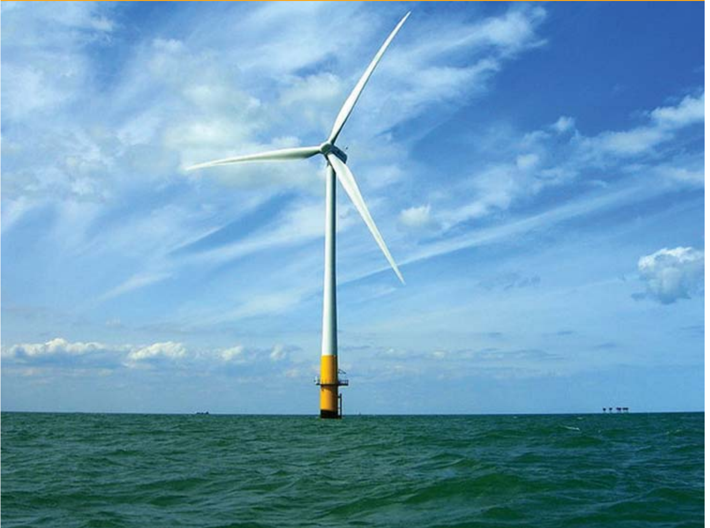
Figure 23.1 This wind turbine in the Thames Estuary in the UK is an example of induction at work. Wind pushes the blades of the turbine, spinning a shaft attached to magnets. The magnets spin around a conductive coil, inducing an electric current in the coil, and eventually feeding the electrical grid. (credit: phault, Flickr)
