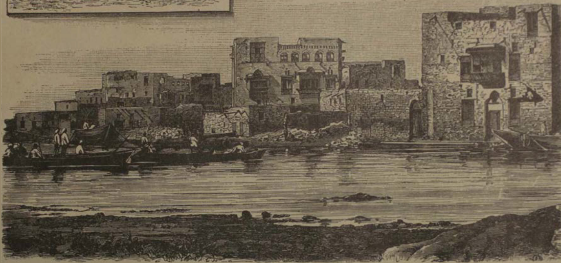
OSMAN DIGNA'S HOUSE IN SUAKIM.
