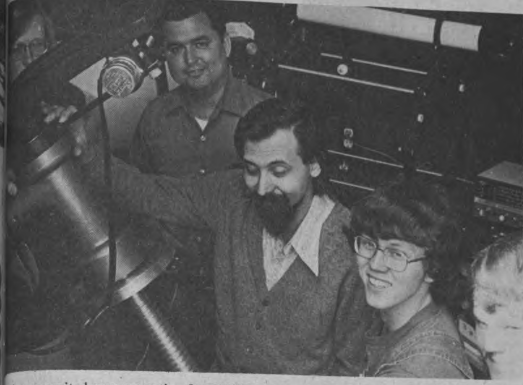
Long awaited new mounting for 12 1/2" telescope in observatory atop Nevins Hall is installed by Dr. Marks, Director of Observatory and Planetarium; Dr. Schreuer, Head Dept. of Physics and Astronomy; Jimmy Westlake; Rob Suggs; Roy Young; Richard Henderson.
