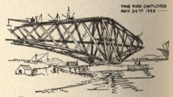
Fig. 25.—How the Forth Bridge was erected.
