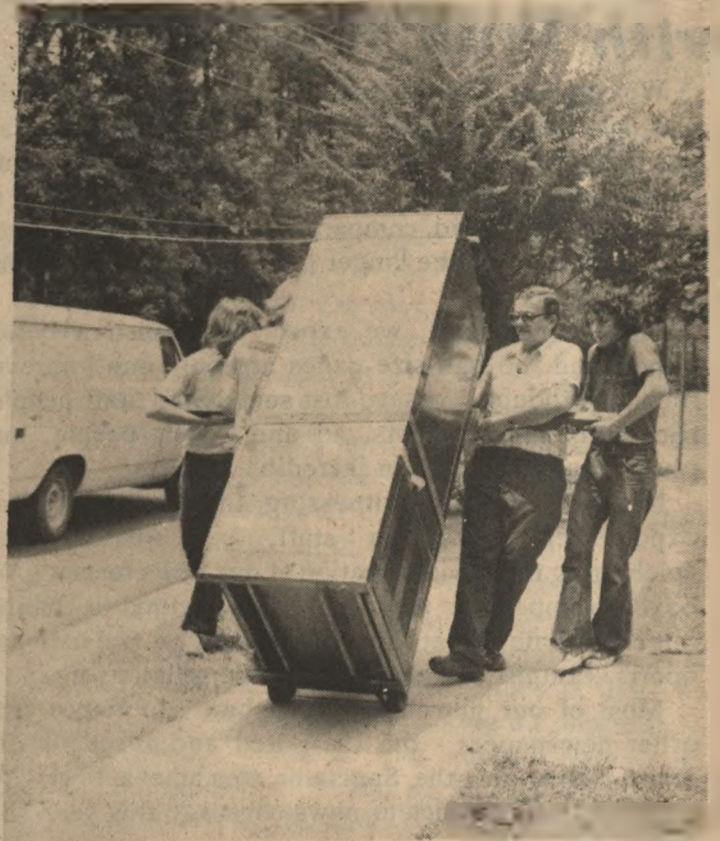
Station Personnel move transmitter to its new home.
