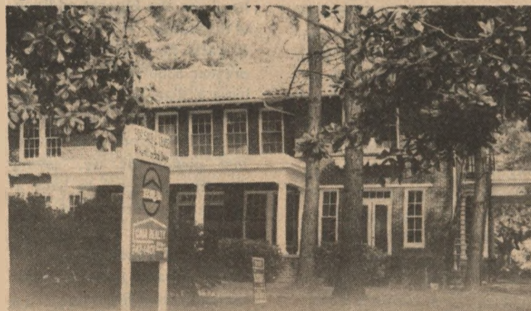
These houses have been bought and restored to their original condition.
