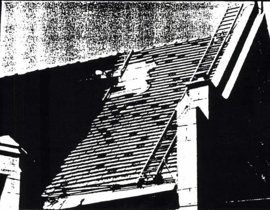
Clay tiles salvaged from less visible areas are being reinstalled on the primary roof over the nave of St. Mary's R.C. Church in Oswego, New York.
