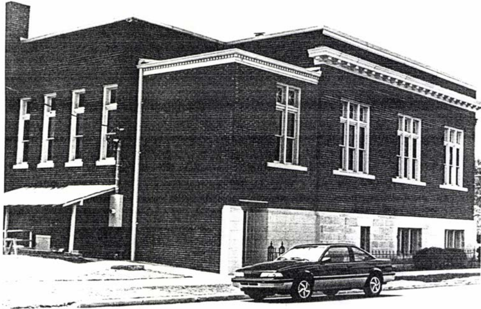
VIEW OF THE REAR ELEVATOR ADDITION ON THE LOWNDES CO. HISTORICAL SOCIETY MUSEUM. ADDITION IS THAT PORTION OF THE BUILDING WHICH HAS A LOWER ROOF.
