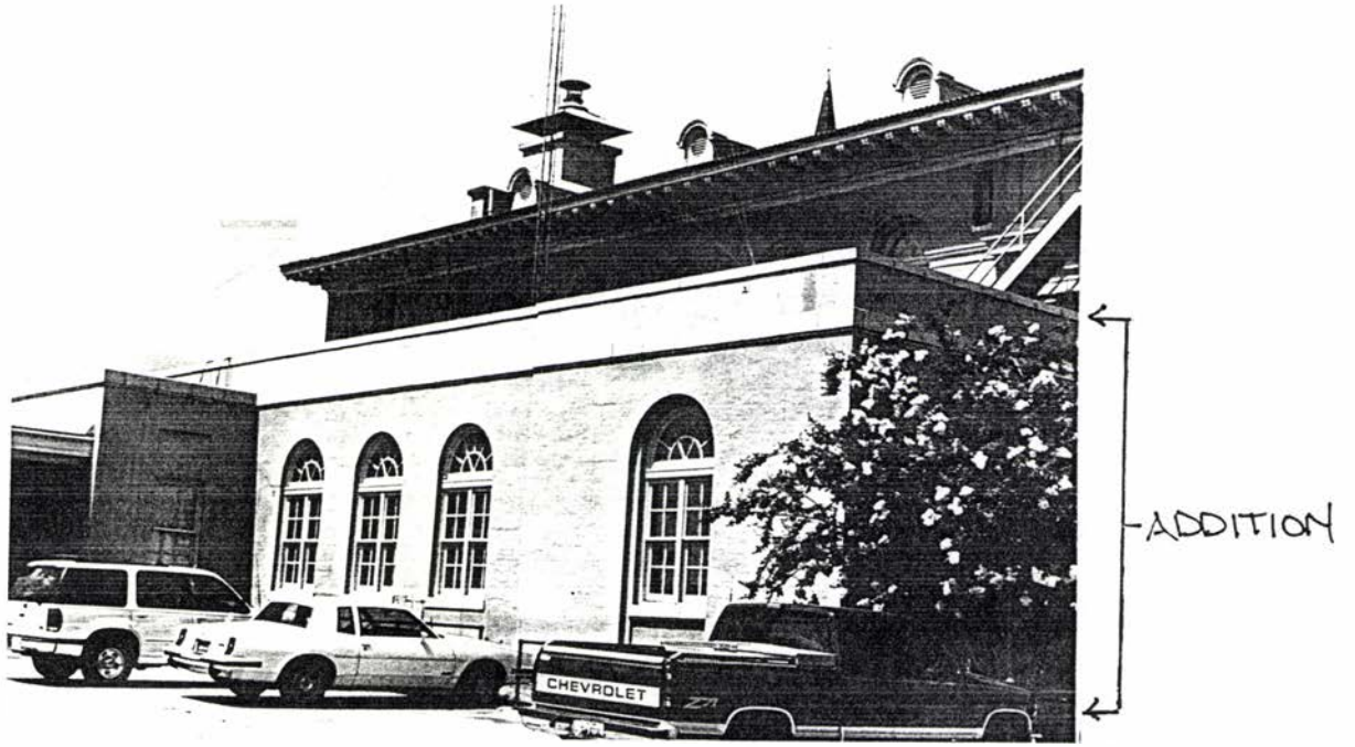
REAR VIEW OF CITY HALL SHOWING ONE-STORY ADDITION
