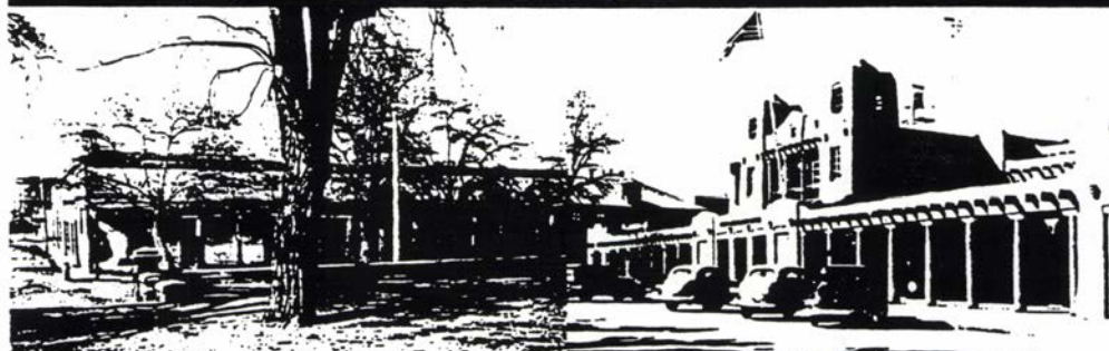
THE WOOD-AND-ADOBE OLD CONVENTO BUILDING ON CATHEDRAL PLACE IN 1911 GAVE WAY TO THE U.S. POST OFFICE, SHOWN HERE CIRCA 1935, CONSTRUCTED OF BRICK VENEERED WITH WOOD AND ADOBE.
