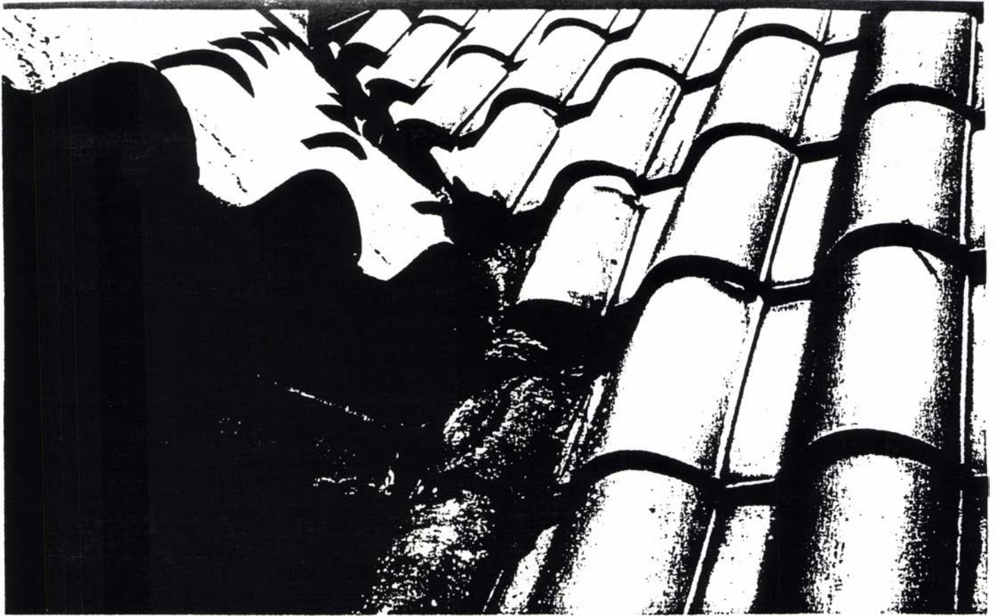
Asphaltic "goop" was slopped on eroded flashing, accelerating corrosion of the metal cornice.
