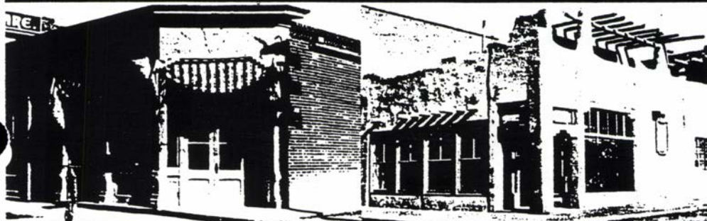
BRICK VENEER COVERED ADOBE ON A CIRCA 1905 MILLENNERY SHOP AT THE CORNER OF WASHINGTON AND SAN FRANCISCO AVENUES, BUT ADOBE PREVAILED ON A TICKET OFFICE AT THE SAME LOCATION IN THE 1920S.
