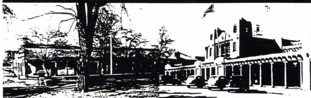
THE WOOD-AND-ADOBE OLD CONVENTO BUILDING ON CATHEDRAL PLACE IN 1911 GAVE WAY TO THE U.S. POST OFFICE, SHOWN HERE CIRCA 1935, CONSTRUCTED OF BRICK VENEERED WITH WOOD AND ADOBE.
