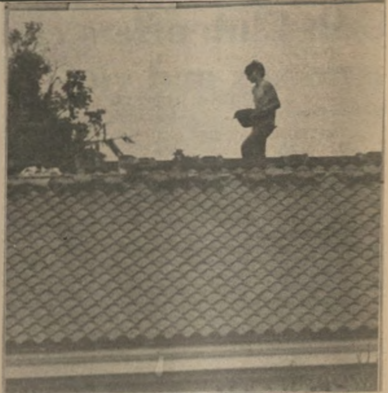
Spring spruce up- Hopper Hall gets fresh, new tar paper.
