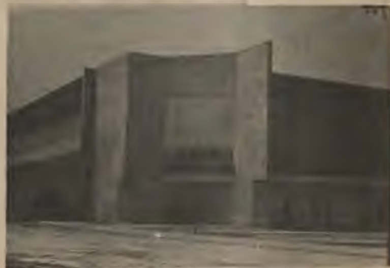
Outside view of new P.E. complex
