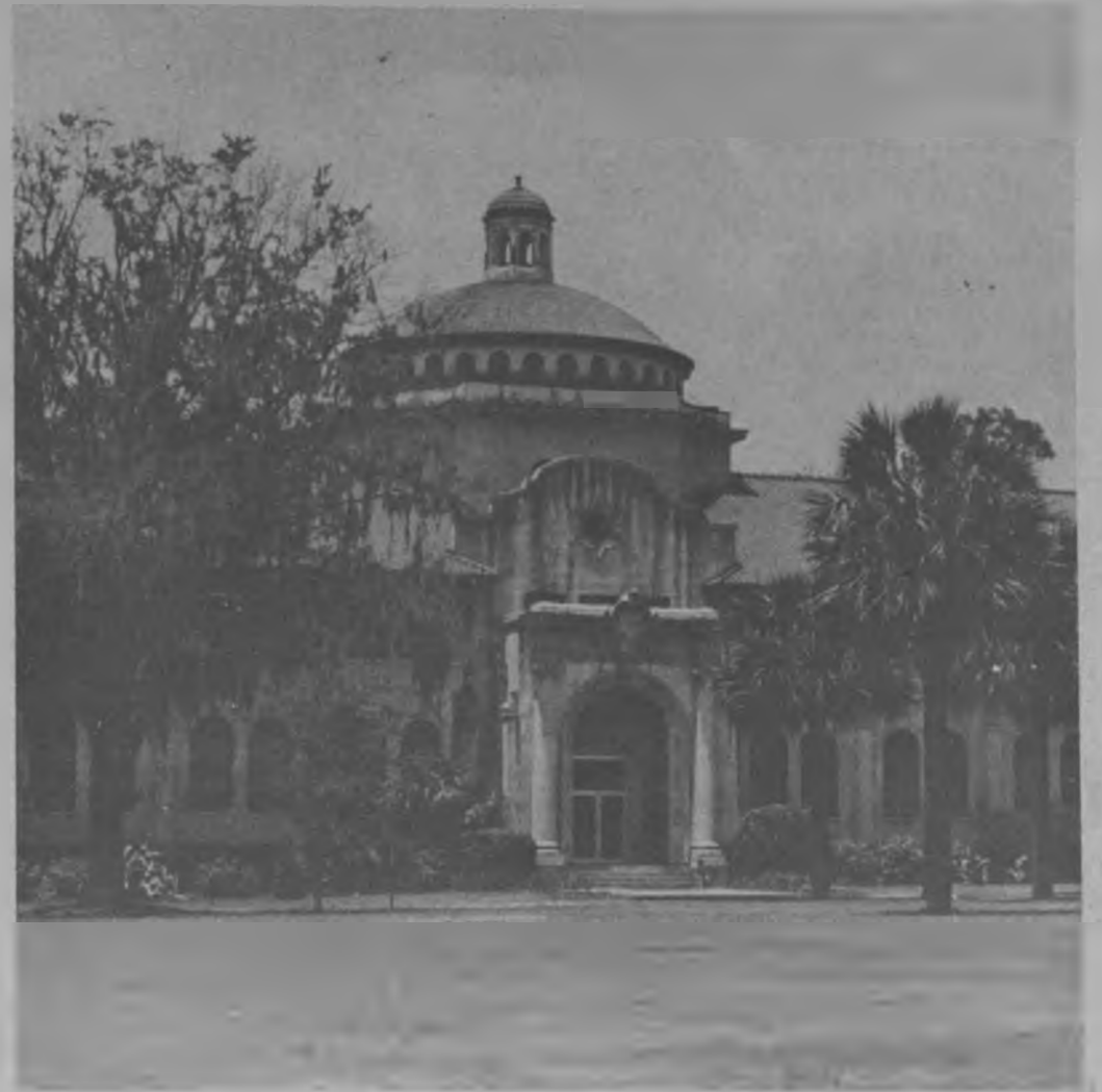
Badly deteriorating West Hall is in need of a $4 million renovation.
