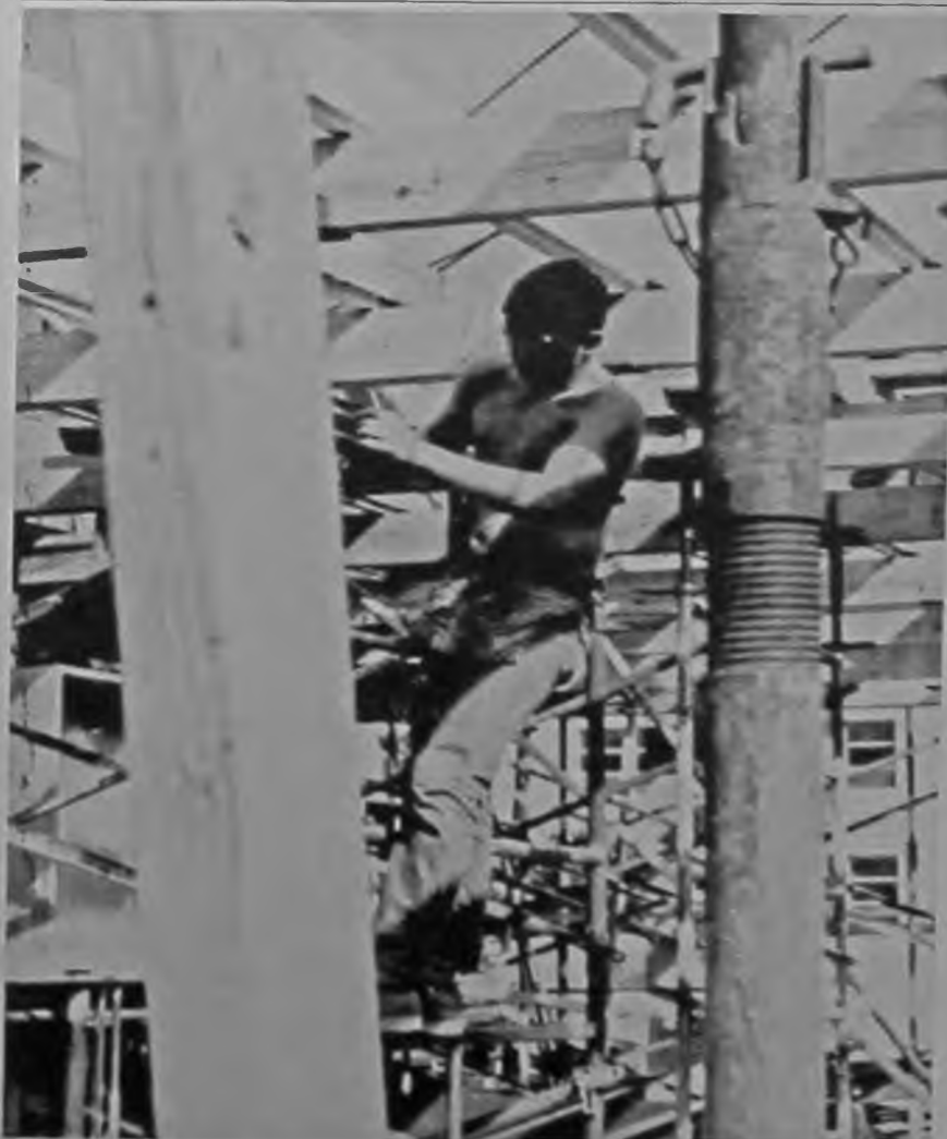
Rising High is the Construction of New Buildings at VSC.
