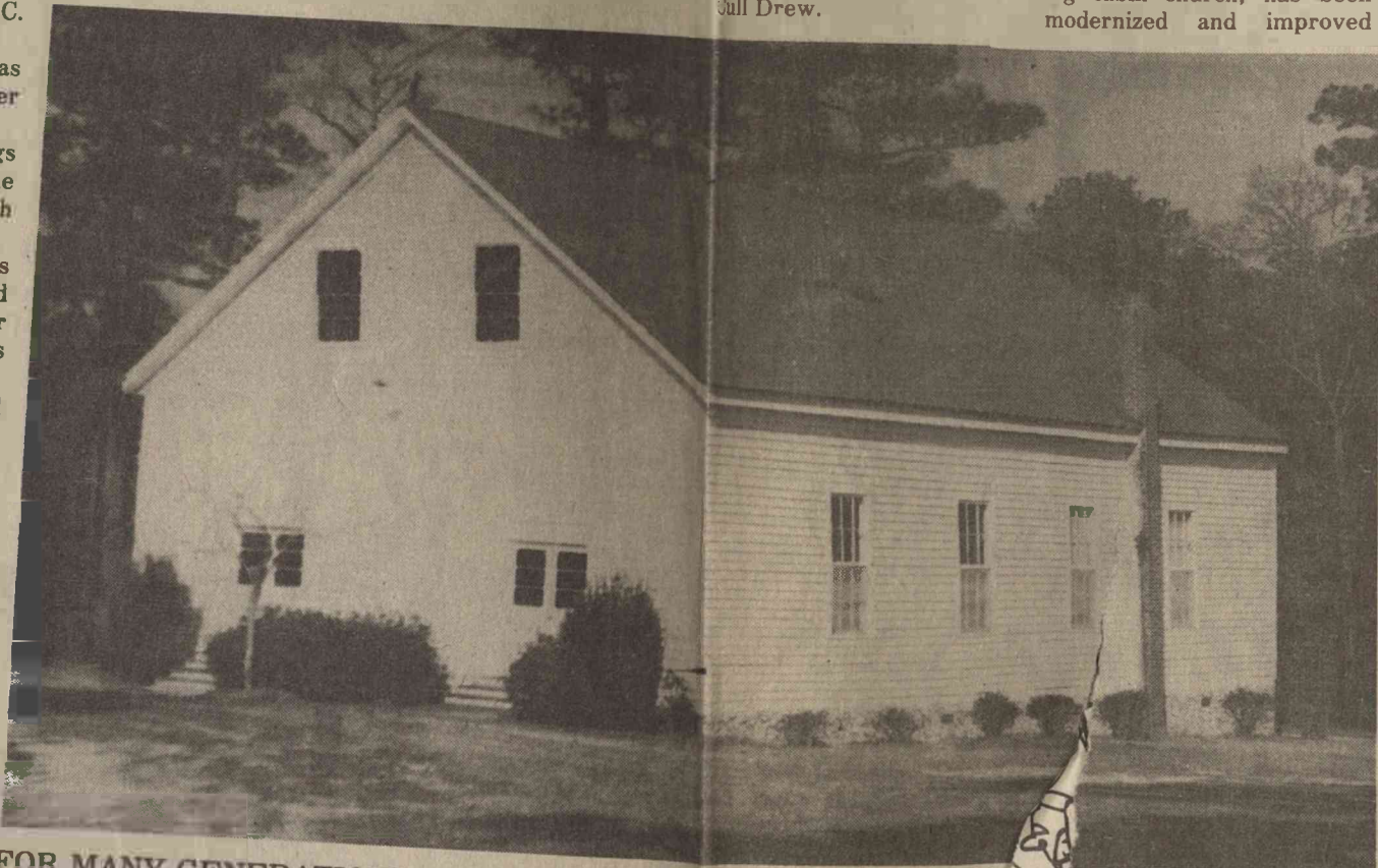
FOR MANY GENERATIONS BOLD SPRINGS UNITED METHODIST CHURCH has stood as the religious and community center of a large section in the eastern part of Grady County. It continues to be a very vital part of Methodism in Grady County. (Photo by Hugh Gandy)
