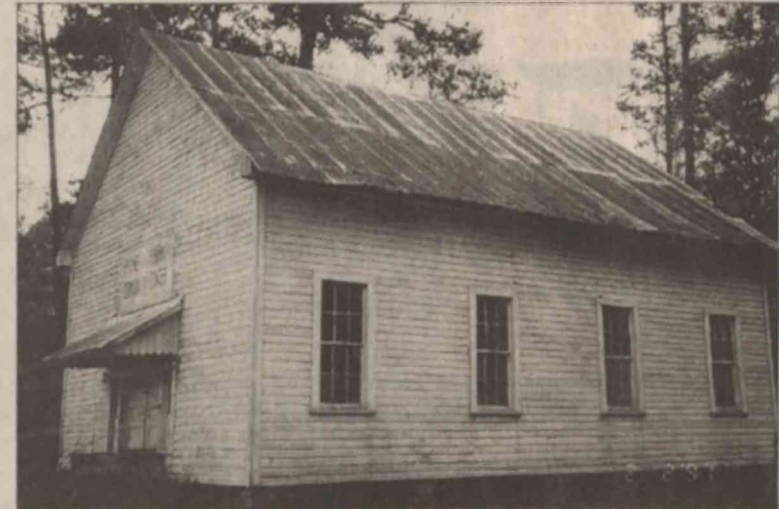
THE PINE PARK COMMUNITY CENTER building stands in the 1997 photo, just before the building fell victim to acts of vandalism and theft.
