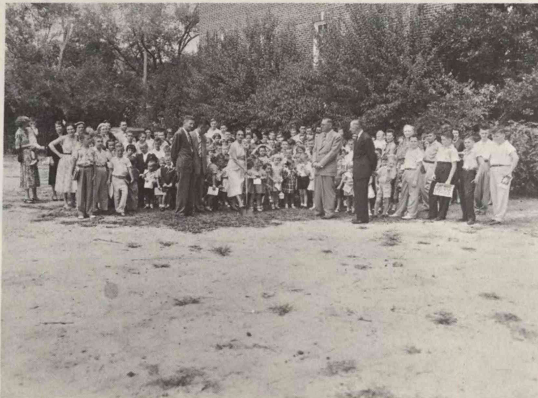
Ground-breaking for Children's Division Building. Second phase of 1952 Expansion Program. Completed in June, 1955, during the pastorate of Rev. L. E. Williams.
