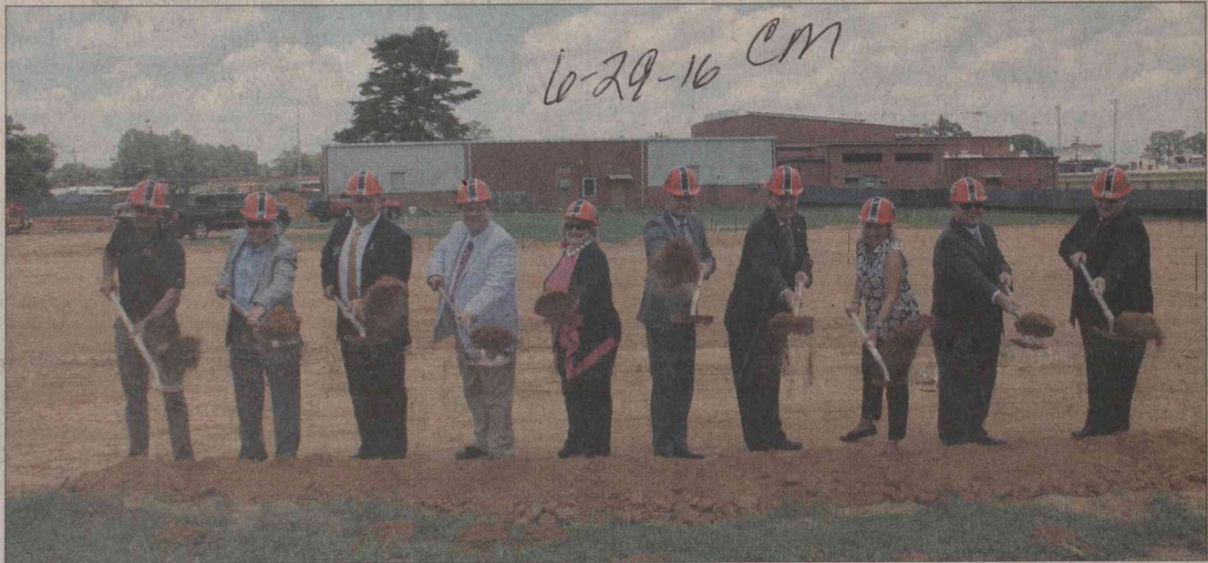
GEORGIA LT. GOV. CASEY CAGLE , center, was joined by general contractor Doug Young of PDC Construction Inc., of Bainbridge, architect Greg Smith, Technical College System Executive Director Mark Peavy, Grady County School Superintendent Dr. Kermit Gilliard, State Representative Darlene Taylor, (Cagle), Senator Dean Burke, Grady County Board of Education Chairman Laura Register, Cairo High School Principal Chris Lokey, and College and Career Academy CEO Todd Gainous in officially breaking ground for the new Cairo High School College and Career Academy last Thursday.
