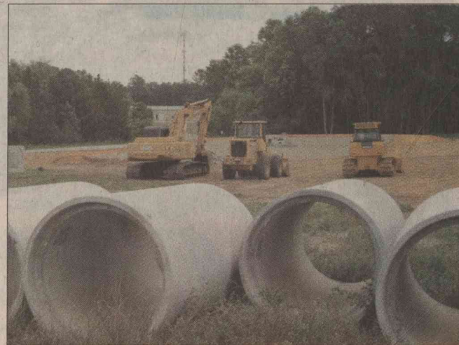
THIS RETENTION POND on the Cairo High School campus was constructed in partnership with the City of Cairo public works department. The new pond will retain storm water from the school's new College and Career Academy facility and release it into the stormwater drainage system. THESE PIPES are yet to be installed that will connect the retention pond to the city's stormwater drainage system.
