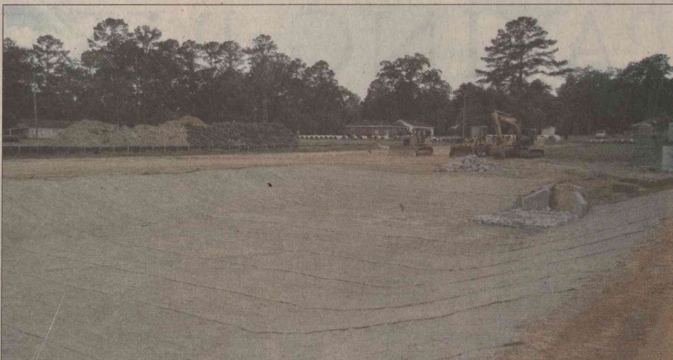
THIS RETENTION POND on the Cairo High School campus was constructed in partnership with the City of Cairo public works department. The new pond will retain storm water from the school's new College and Career Academy facility and release it into the stormwater drainage system. THESE PIPES are yet to be installed that will connect the retention pond to the city's stormwater drainage system.
