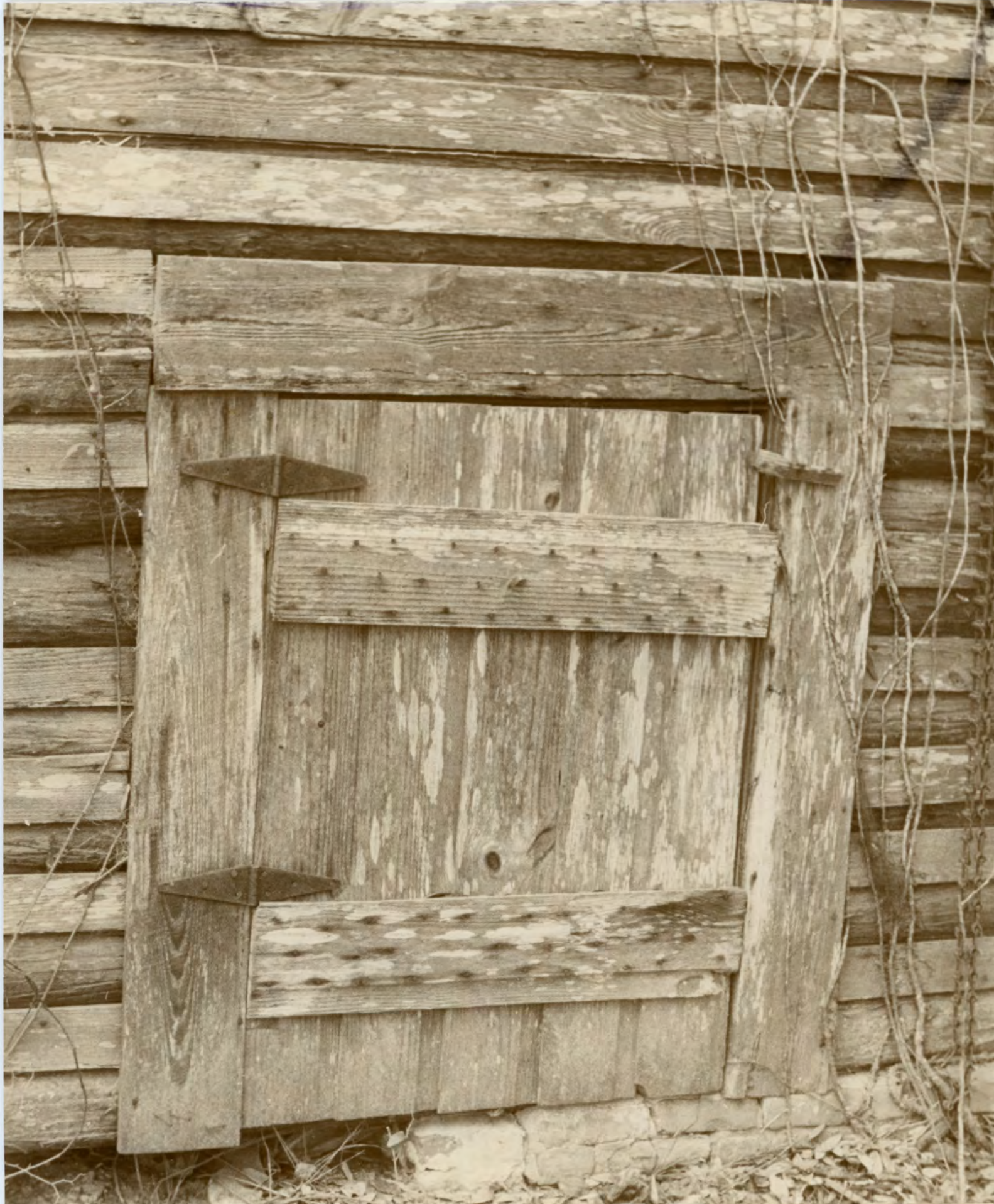
This picture shows the door of a log tobacco barn. The log barn has logs on the inside of the door for insulation.
