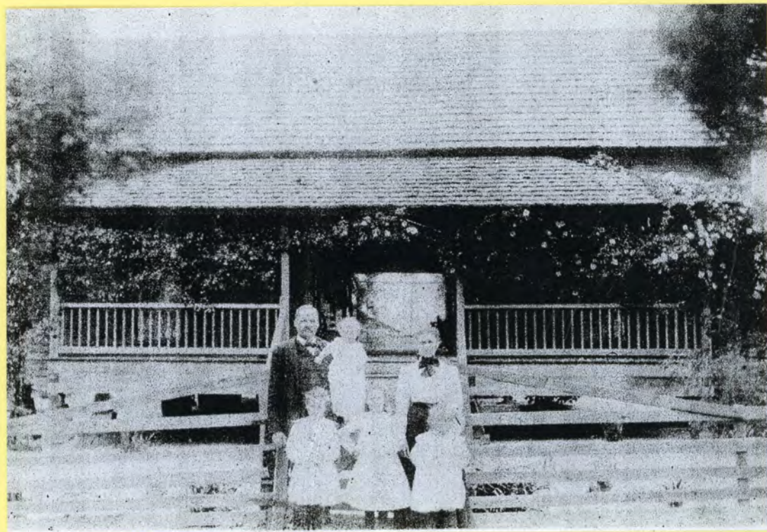
JOHN MORRISON HOME, ABOUT 1900 This home, now gone, had the dogtrot hallway and wide vine shaded porch often found before air conditioning. Johnson of Angus, married Mary Etta Ingram. Their daughters were students at Union School and at Morven School after the Union schoolhouse burned. They hired a music teacher to live in the home to provide lessons for their girls and neighbors.
