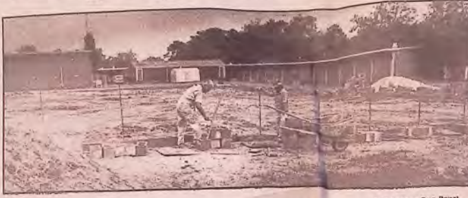
Construction workers in process of rebuilding Whigham High gymnasium
