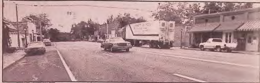
Broad Street — U.S. 84 — five-laning completed in Whigham downtown
