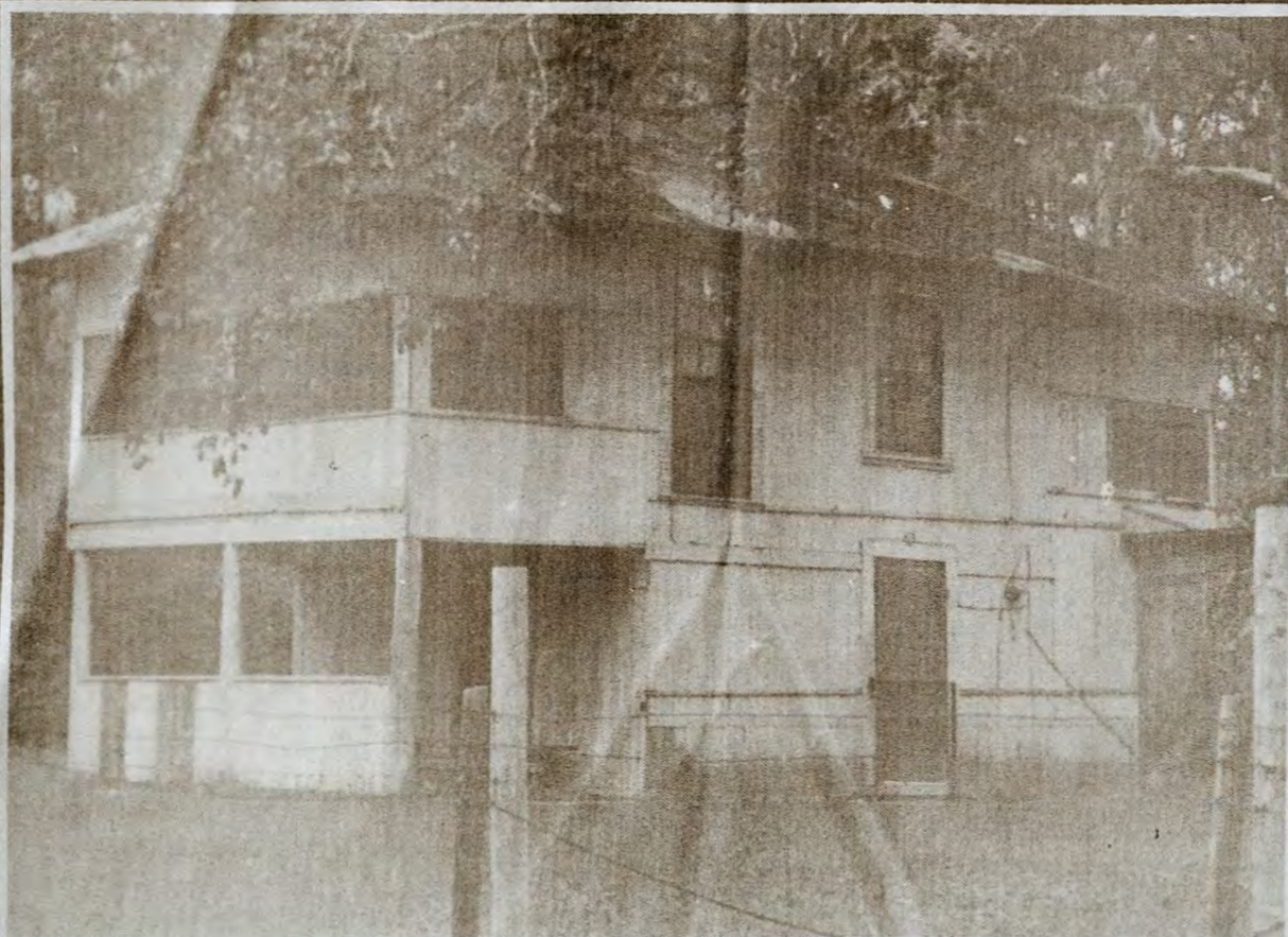
Pictured is a cottage at the Blue Springs entrance which has been restored by owner Walter Cunningham.
